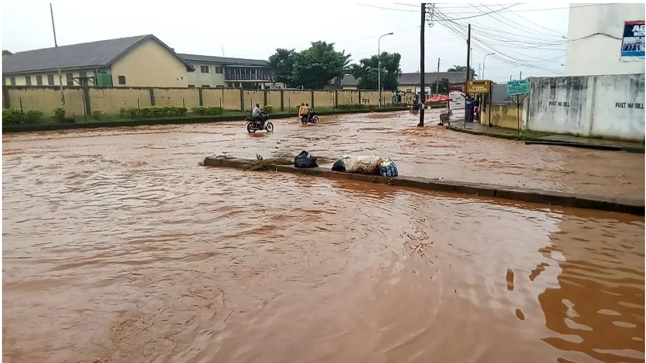
Fig. 1.6: Flooding at EFAB Estate, Lokogoma, Abuja, 2019.
